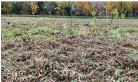
6. Placement of the supporting pole
