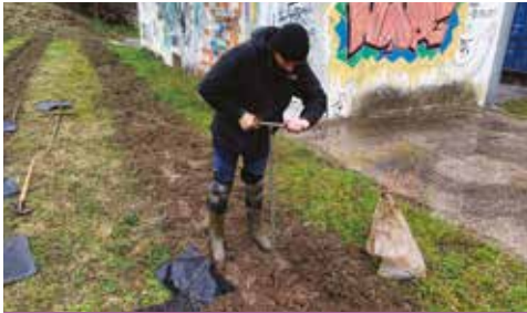
2. Excavation of the hole using manual mechanical equipment or a motorised auger
